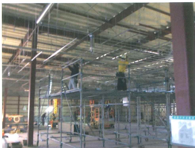
軽量下地施工
